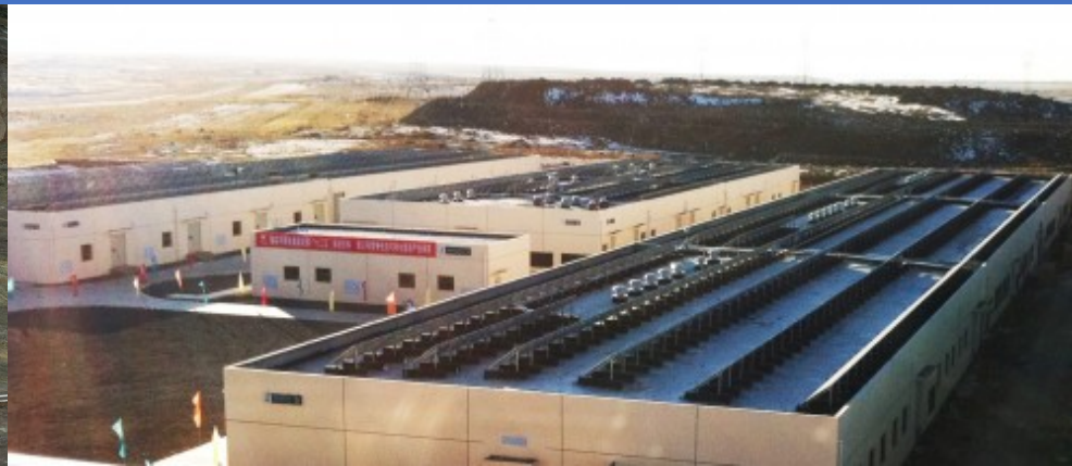
BYD-State Grid Battery ES Array in Zhangbei
