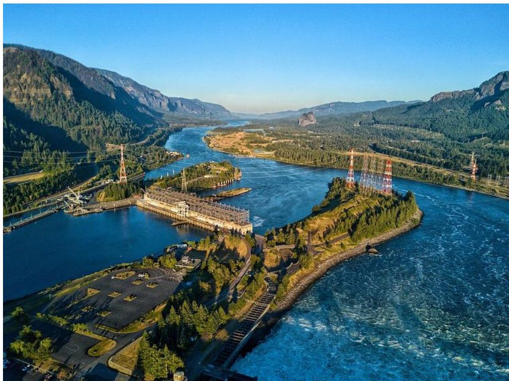
Figure 10: The Bonneville Dam in Washington, first opened in 1937, can provide over 1.2 GW of power. 143 Image courtesy of the U.S. Department of Energy. 144
