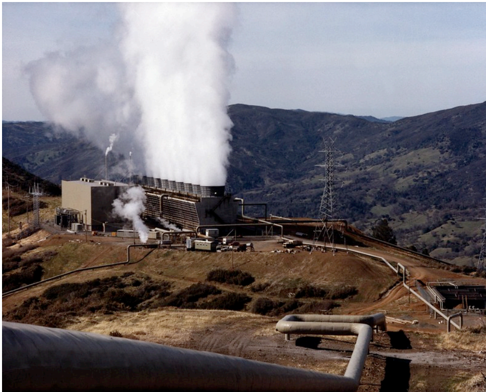
Figure 6: The Geysers complex in northern California comprises 18 geothermal power plants providing over 900 MW of electricity. Image courtesy of the U.S. Department of Energy. 100
