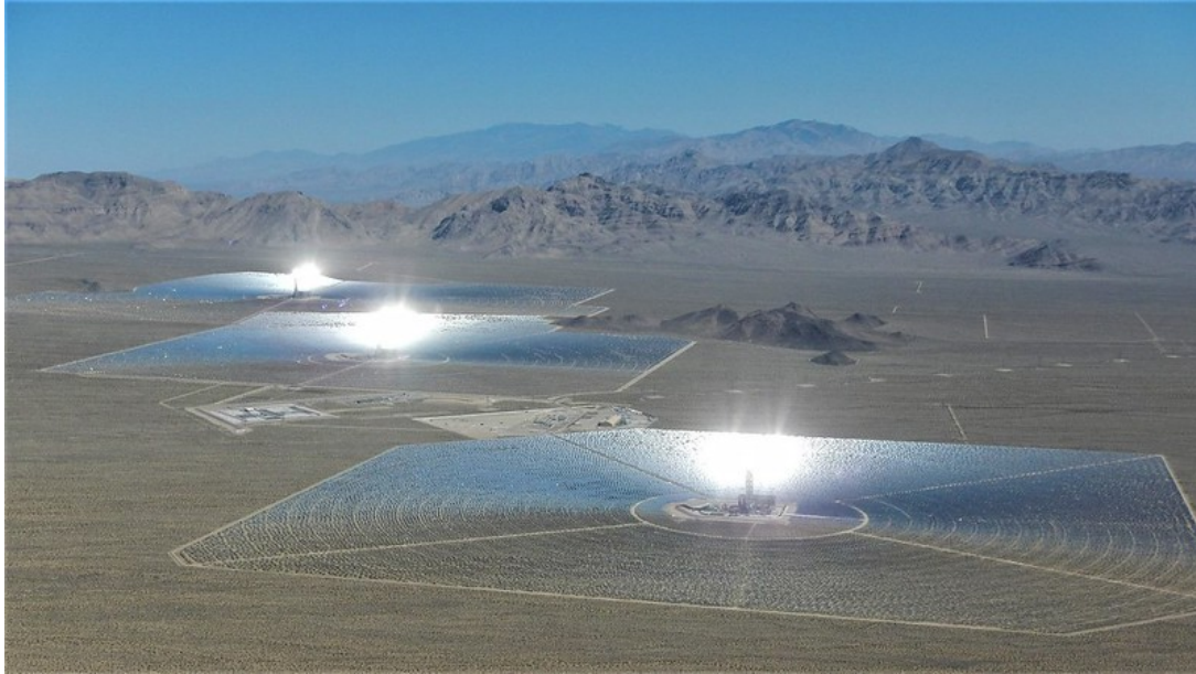
Figure 8: The Ivanpah Solar Electric Generating System in the Mojave Desert produces 392 MW power. Image courtesy of the U.S. Department of Energy. 117
